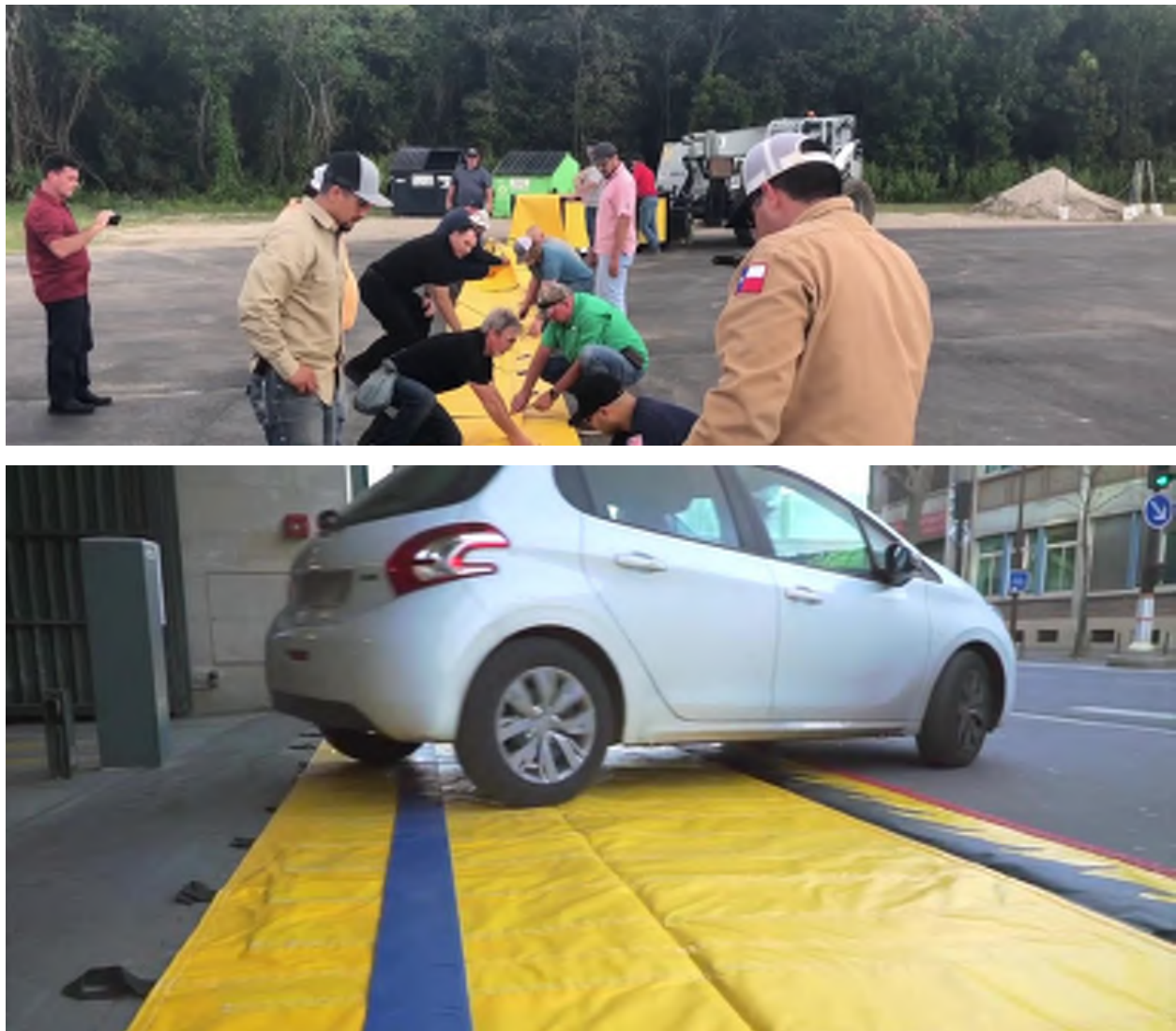
Figure 3-2: Temporary Flood Barrier - Deployment
