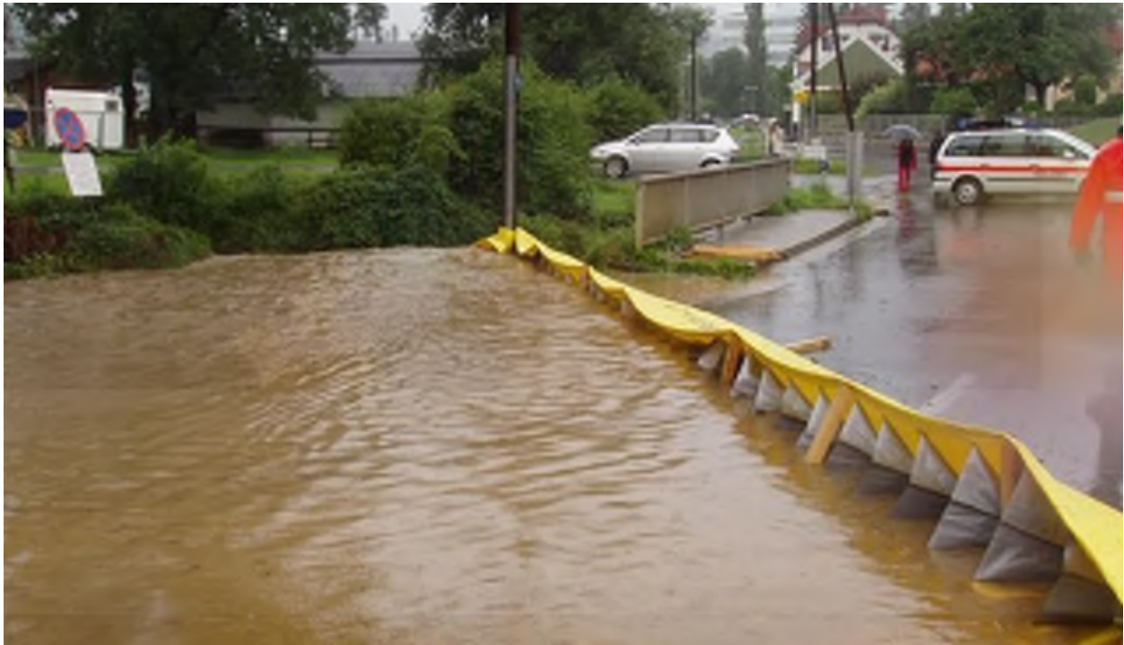
Figure 3-3: Temporary Flood Barrier – Rising Flood Water
