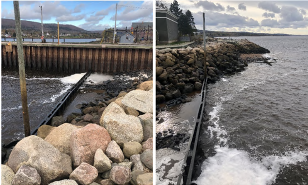
Figure 3-6: Existing Condition at King's Wharf
