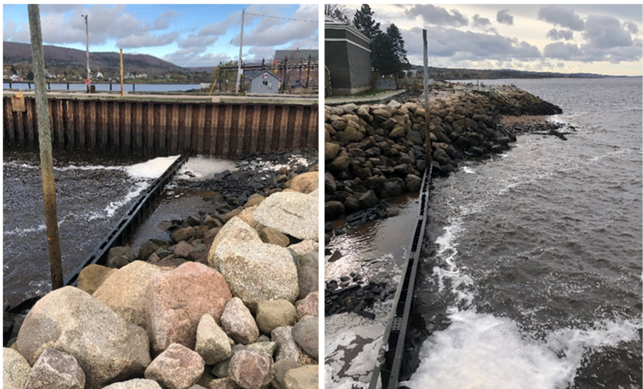
Figure 3-6: Existing Condition at Town Wharf
