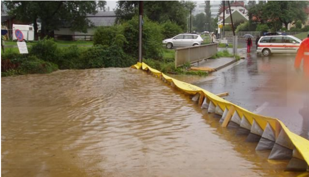
Figure 3-3: Temporary Flood Barrier – Rising Flood Water
