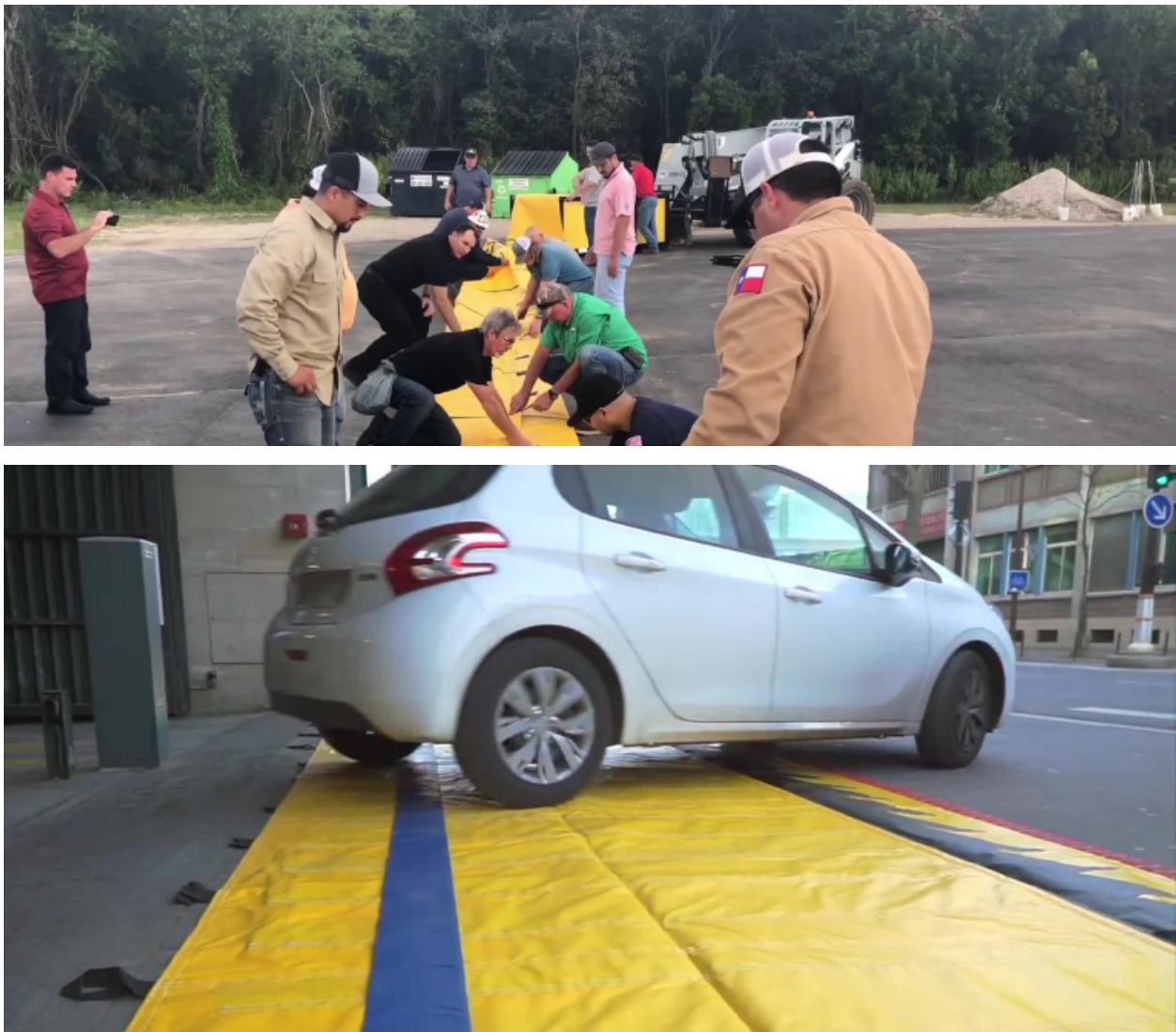
Figure 3-2: Temporary Flood Barrier - Deployment
