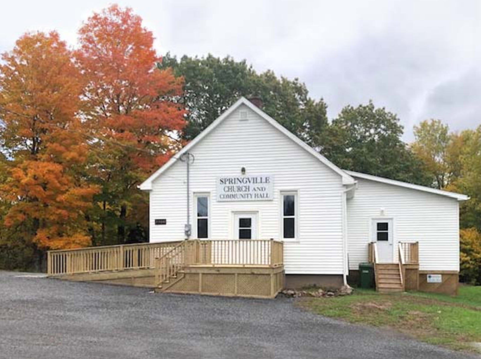
Springville Church and Community Hall, Springville
