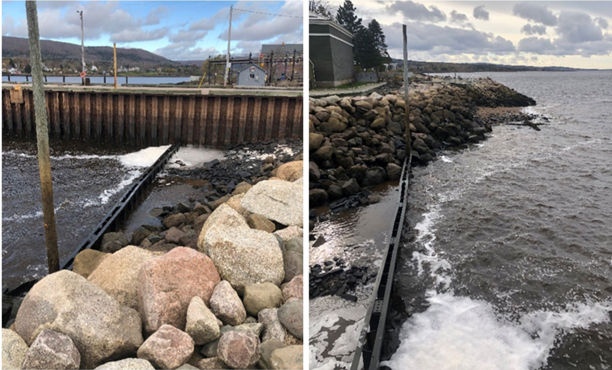
Figure 3-6: Existing Condition at Town Wharf
