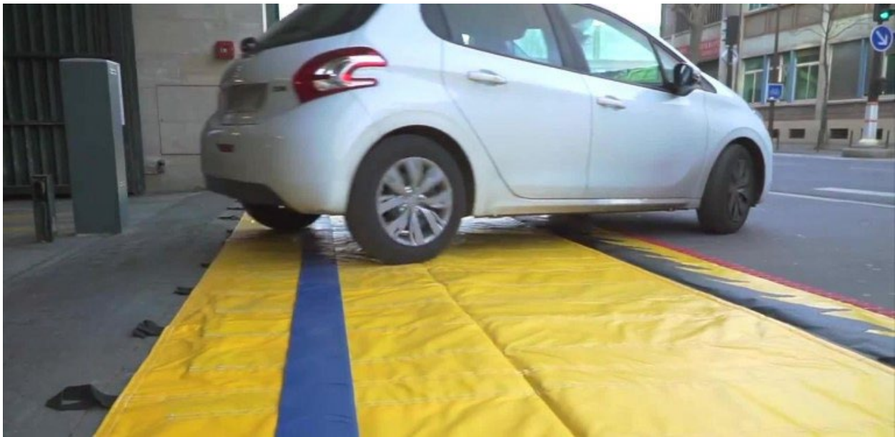
Figure 3-2: Temporary Flood Barrier - Deployment
