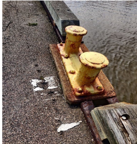
Figure 10 - Steel Bollards Anchored in Concrete
