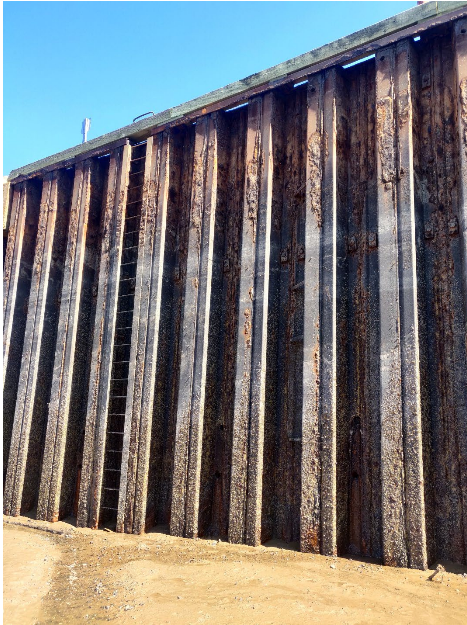
West Side of Wharf Showing Drainage Holes Near Bottom of Piling
