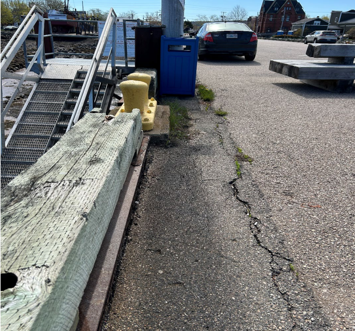
Top of Ramp to Floating Dock
