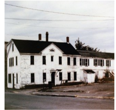
Sinclair Inn before restoration c1980
