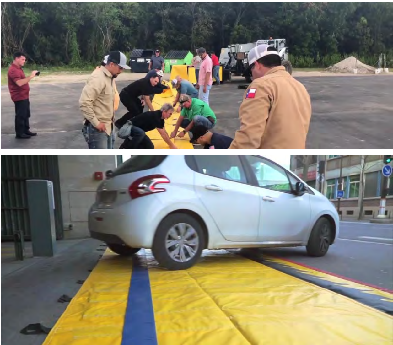
Figure 3-2: Temporary Flood Barrier - Deployment
