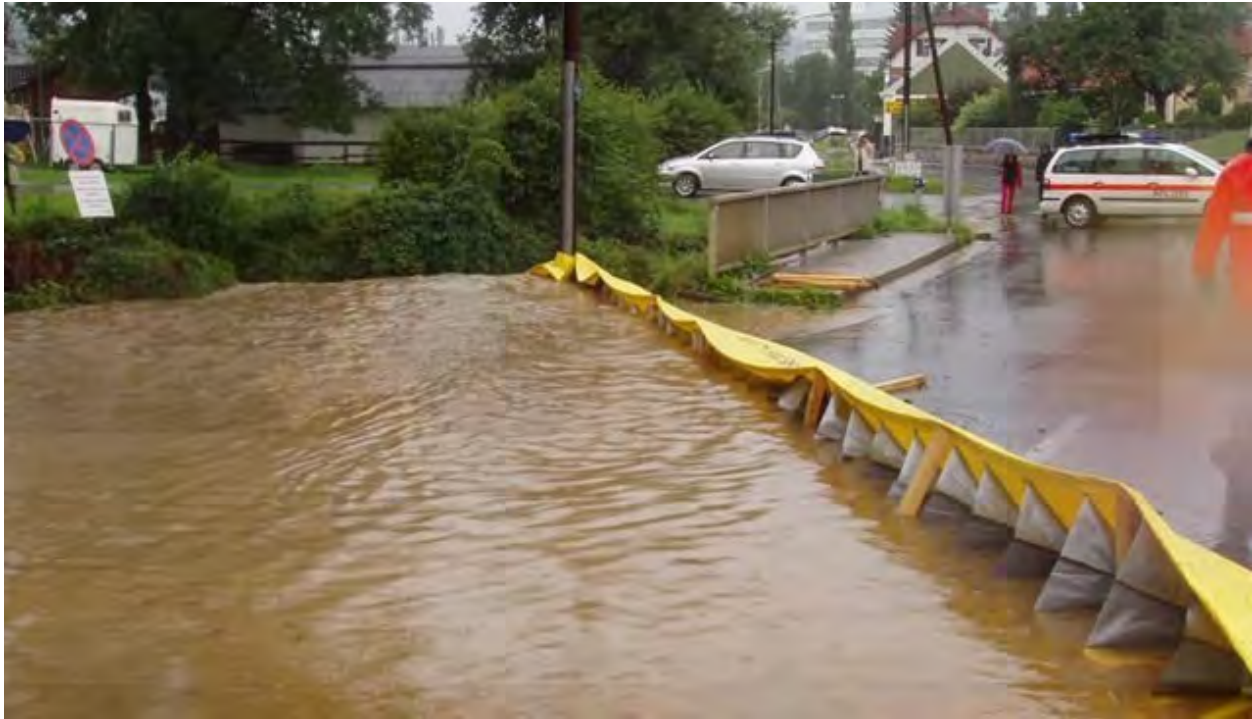
Figure 3-3: Temporary Flood Barrier – Rising Flood Water
