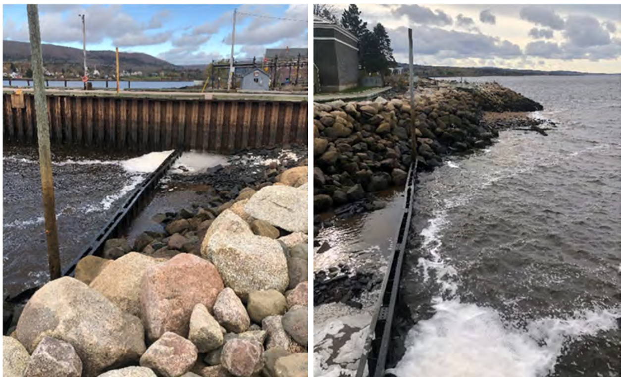
Figure 3-6: Existing Condition at Town Wharf
