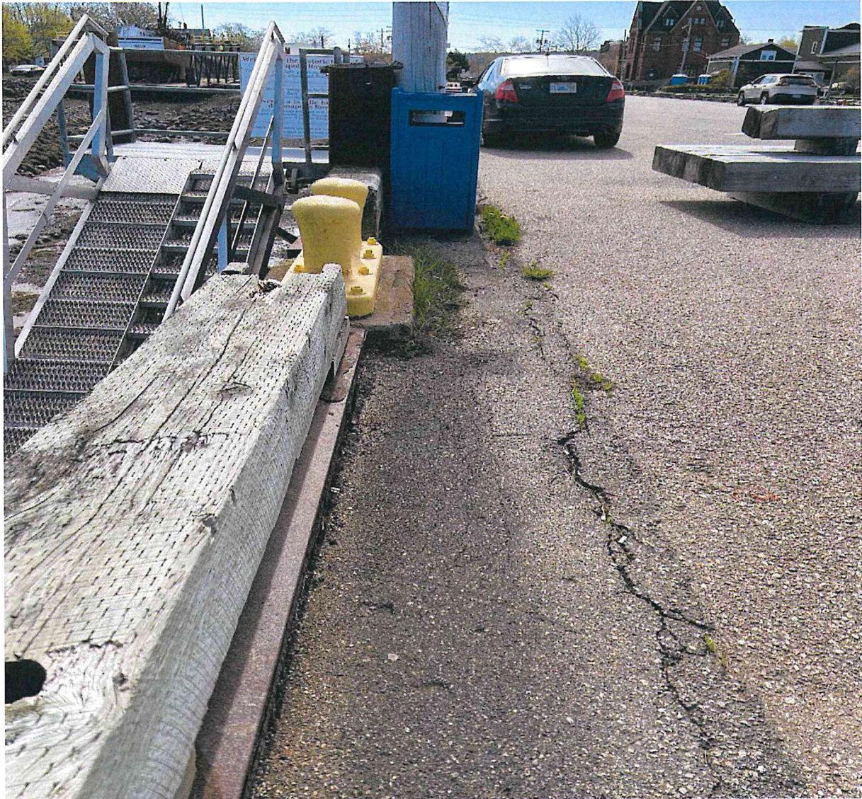
Top of Ramp to Floating Dock
