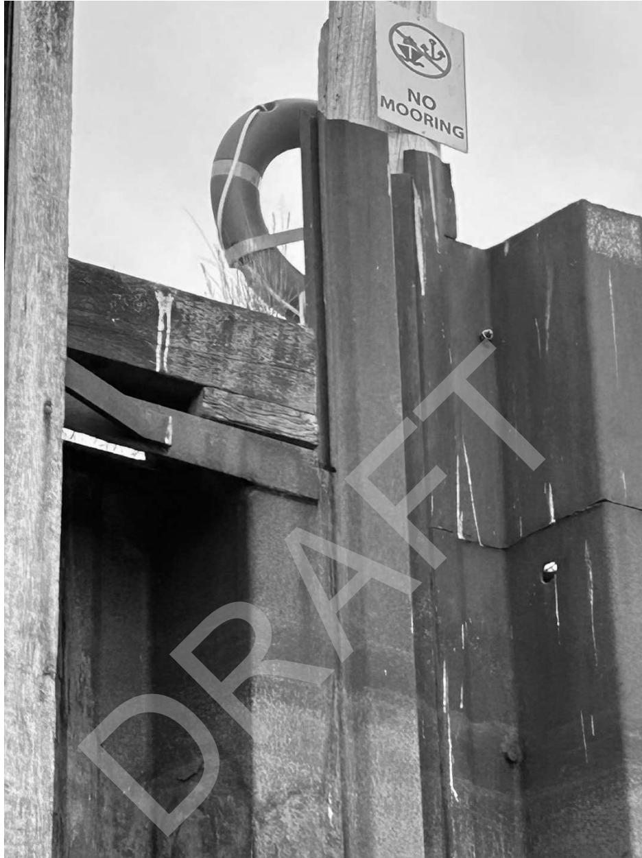
New signage limiting use and safety throw ring on wharf
