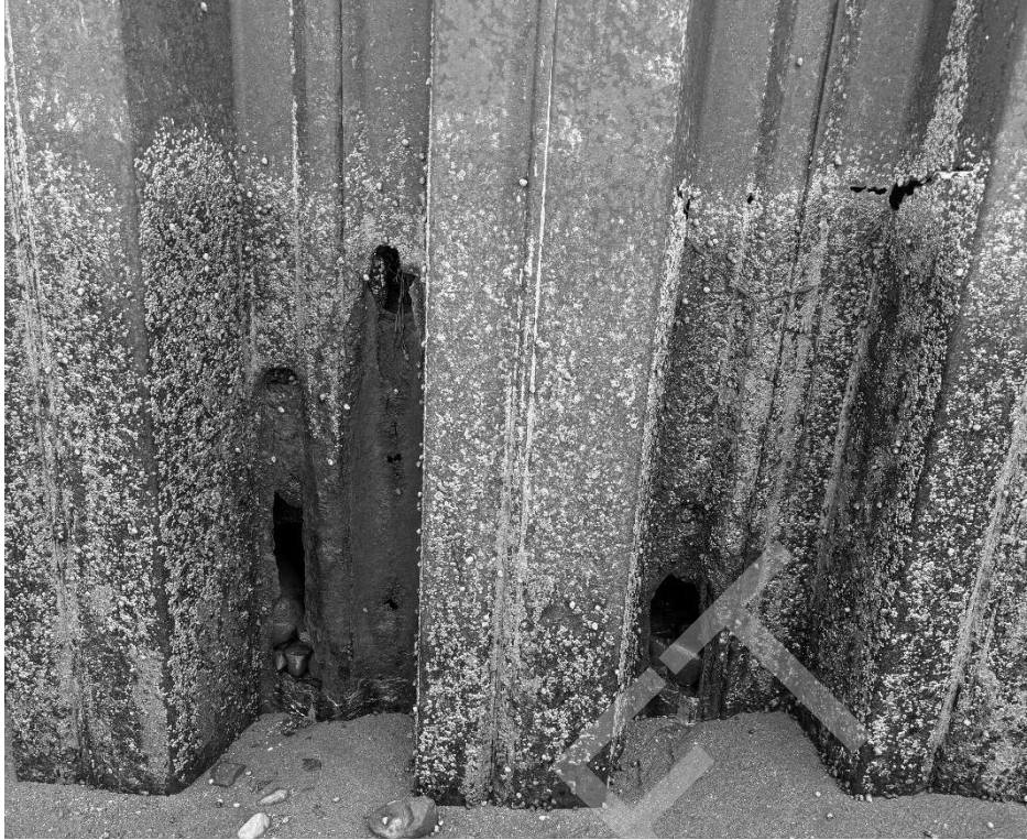
West side of wharf also rusting away near bottom note some rock ballast gone.
