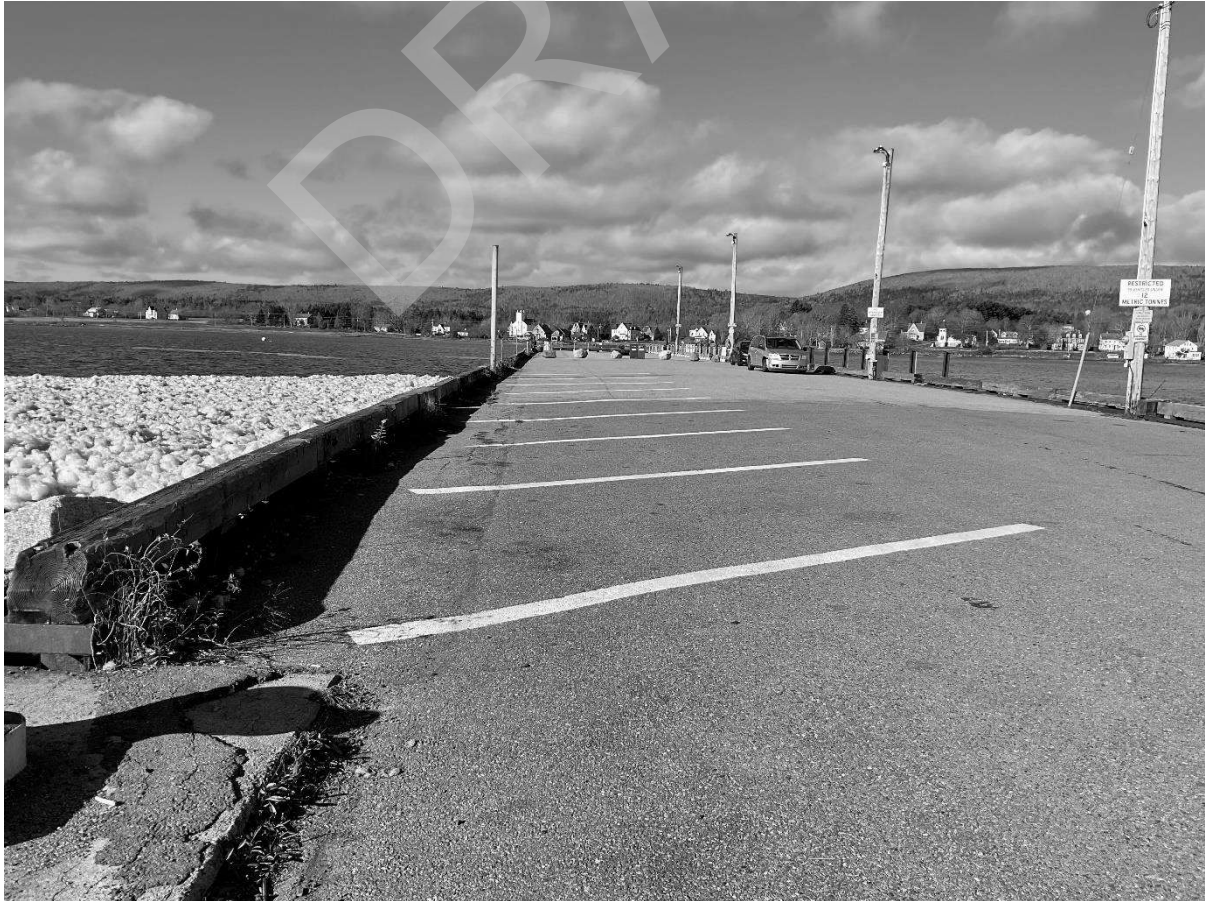
Existing Parking spots 10 spots.
