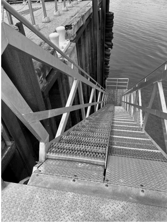
Figure 8 – Floating dock with aluminum ramp/stairs.
