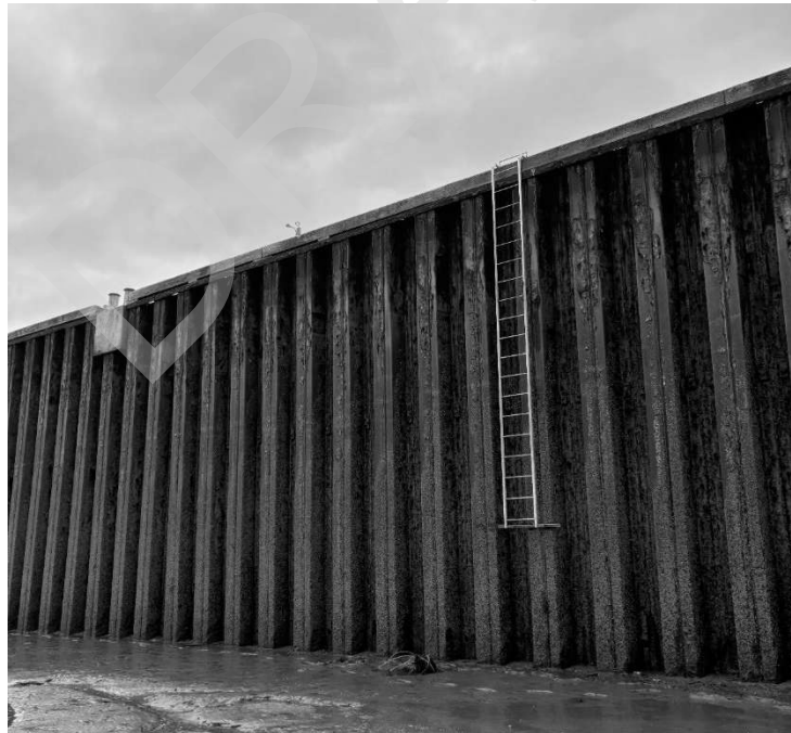
Figure 10 – Portable aluminum ladder in good condition (West Side).
