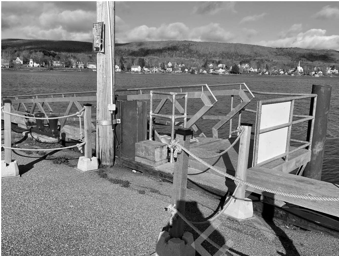
Floating Dock Access from Wharf
